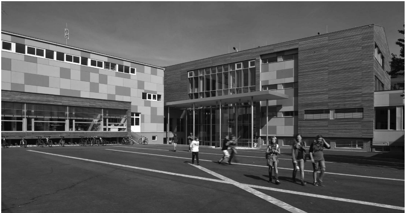
School entrance after renovation [ARCH+MORE/ Blende 16]
